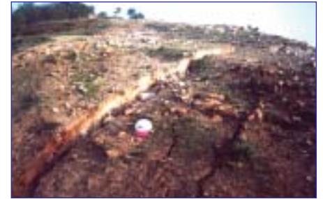
Figure 5: Landslide with cracks in Ait Daoud area
